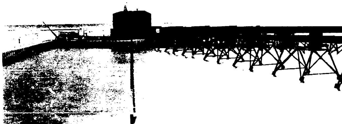
Figure 2. Surface detonation cab, showing pipe array for diagnostic experiments, REDWING.
